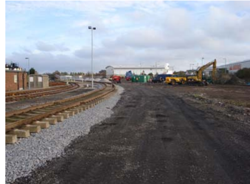
Fratton Goods Yard during refurbishment looking north
